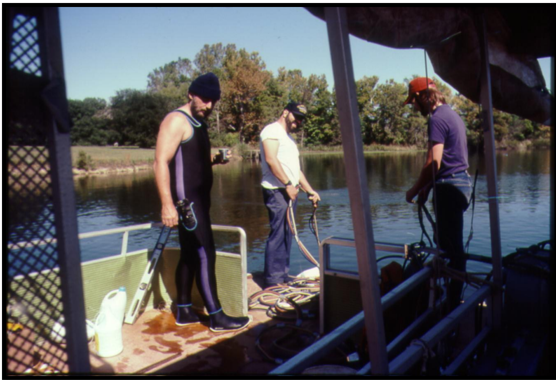
Figure 10: Surface tenders paying out air/communications lines.
