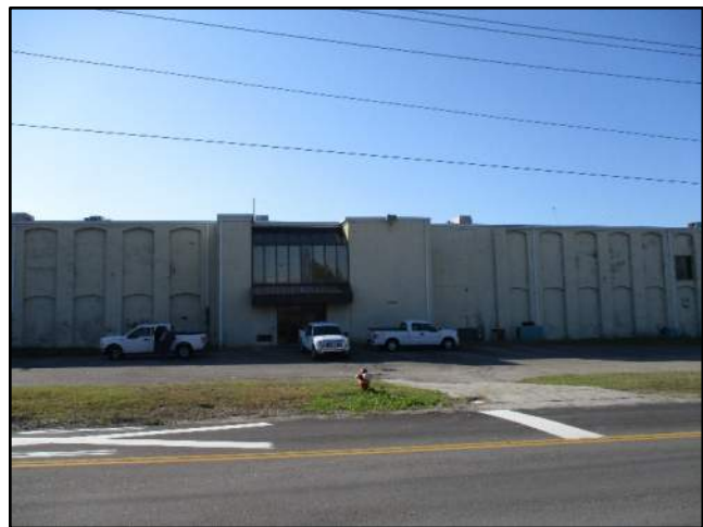
Photo 1. University of South Carolina, former SCE&G Compound, Main Building (Building 1) located at 1206 Flora Street, Columbia SC.
