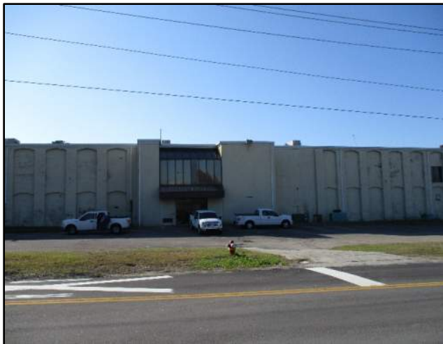
Photo 1. University of South Carolina, former SCE&G Compound, Main Building (Building 1) located at 1206 Flora Street, Columbia SC.
