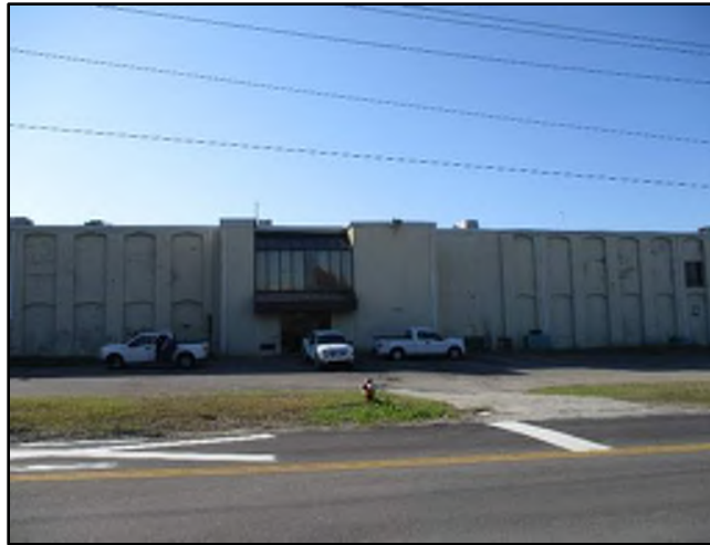
Photo 1. University of South Carolina, former SCE&G Compound, Main Building (Building 1) located at 1206 Flora Street, Columbia SC.
