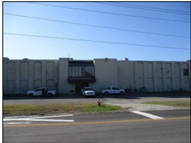
Photo 1. University of South Carolina, former SCE&G Compound, Main Building (Building 1) located at 1206 Flora Street, Columbia SC.
