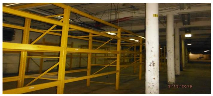
Photo in main warehouse area (Room 100) of the wood columns and metal yellow shelving that contain lead based paint.
