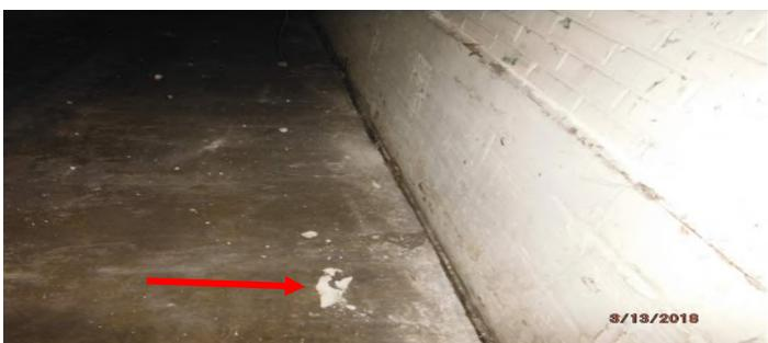
Photo in main warehouse area (Room 100) of the lead-based painted brick walls with photo of paint chips on the floor.
