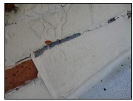
HA-7 – Black flashing mastic (50 SF) Asbestos-containing black mastic was found on flashing at the interface of the exterior wall of the original structure and the metal roof above the rear-loading dock. This material is in good, intact non-friable condition. This material must be removed and disposed of as ACM by a licensed abatement contractor prior to the beginning of renovation activities.
