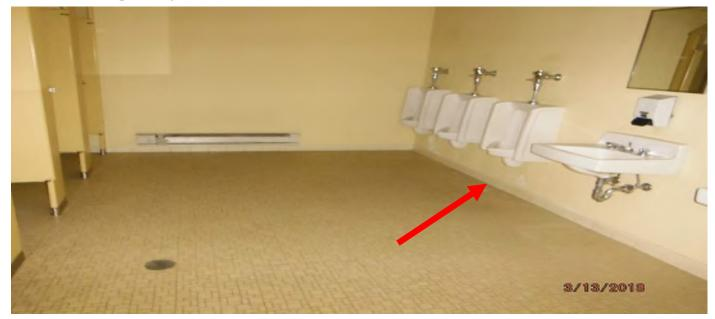
Photo of lead containing tan ceramic baseboard tile, located in bathrooms.
