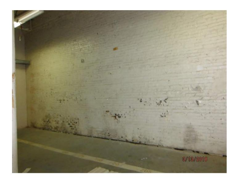
Photo of white painted brick walls painted with lead-based paint located in room 111.
