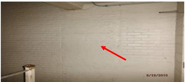
Photo of yellow painted brick walls painted with lead-based paint above drop ceiling on second floor in hallway by stairway STO2.
