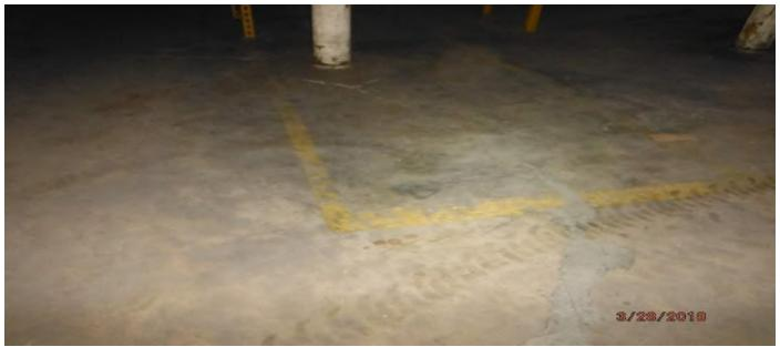
Photo in main warehouse area (Room 100) of the lead containing yellow paint striping on concrete floor.
