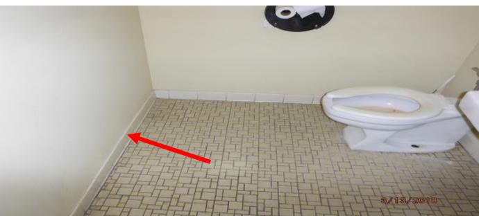
Photo of leadcontaining tan ceramic baseboard tile, located in janitor closet and bathrooms.
