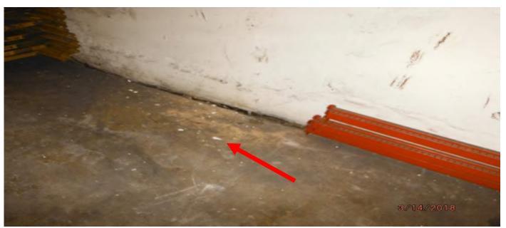
Photo in main warehouse area (Room 100) of the lead-based painted plaster walls with photo of paint chips on the floor.
