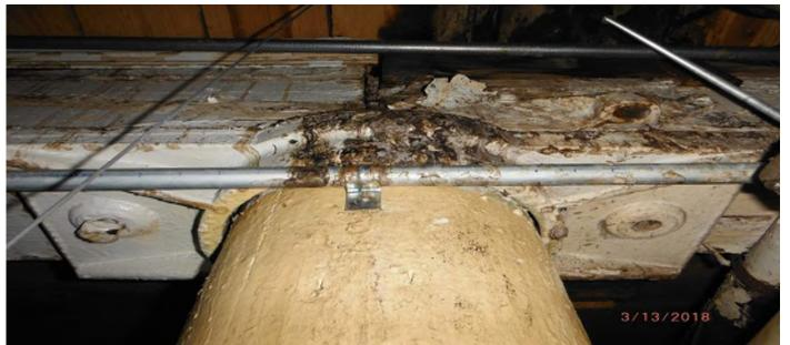
Photo taken from above drop ceiling in room 200 showing wood columns and column top plate that contain lead-based paint. Close-up view of column and column top plate.
