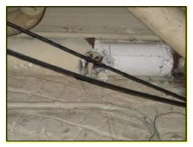
HA-4 – Mudded elbows (2 elbows) The two mudded elbows were found in the north west corner of Room 100 on the 1<sup>st</sup> floor. No other mudded elbows were identified during the field investigation. This material is in an intact but friable condition with only minor localized damage. This material must be removed and disposed of as ACM by a licensed abatement contractor prior to the beginning of renovation activities.
