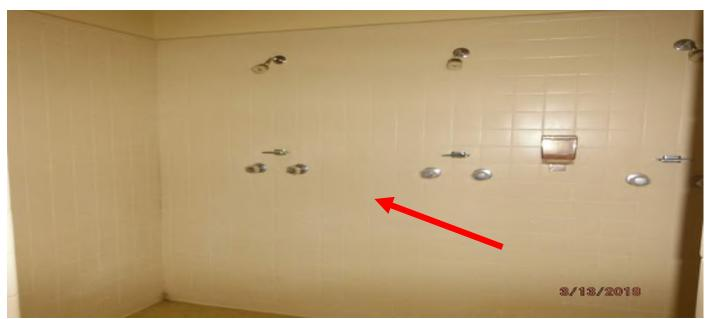
Photo of leadcontaining tan ceramic wall tile located in shower. (Room 238A)
