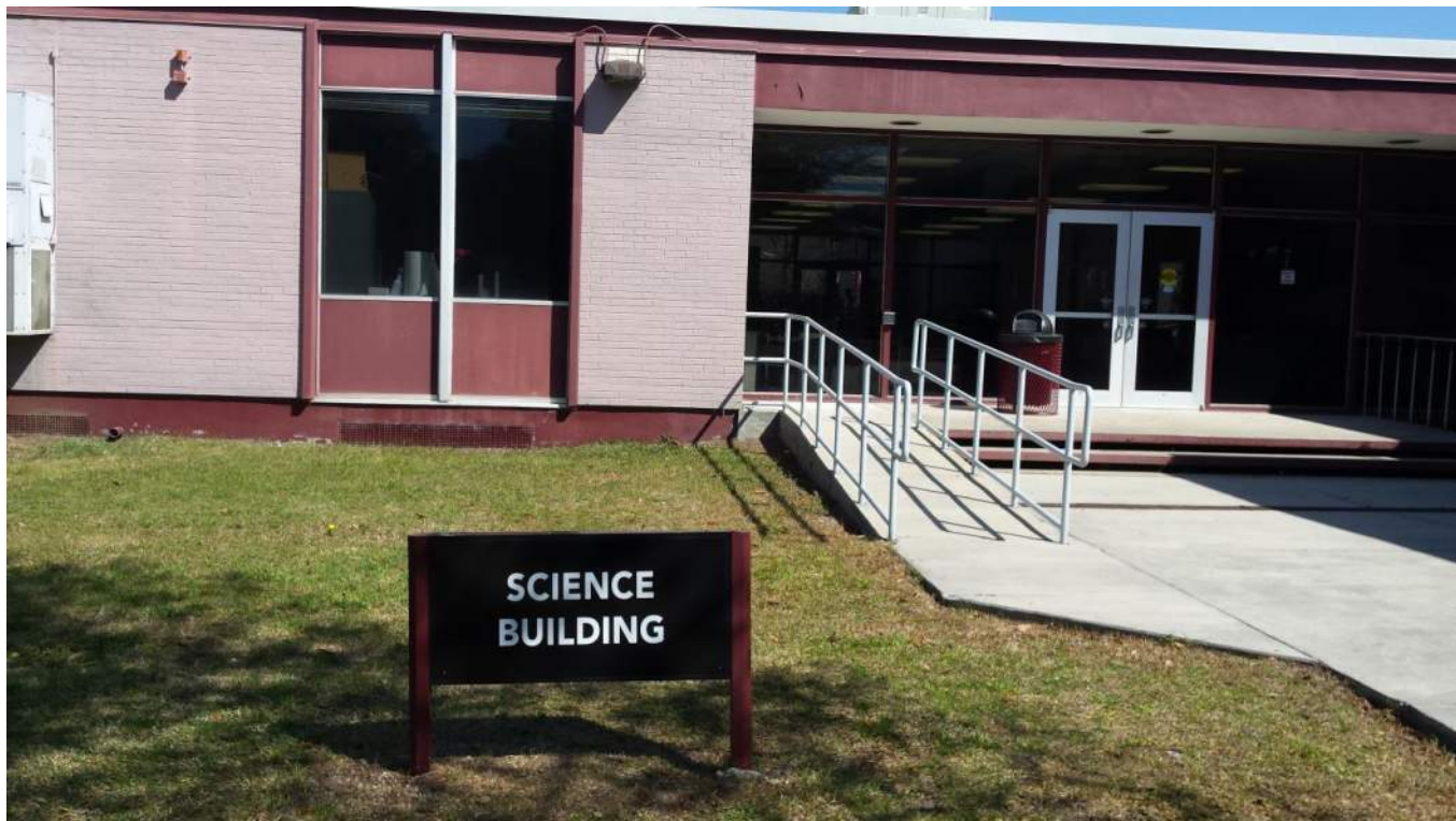
Photograph 1 – View of the USC Science building at 200 Miller Road in Sumter, SC where a Limited Asbestos and Lead Based Paint Survey was performed by ARM Environmental.
