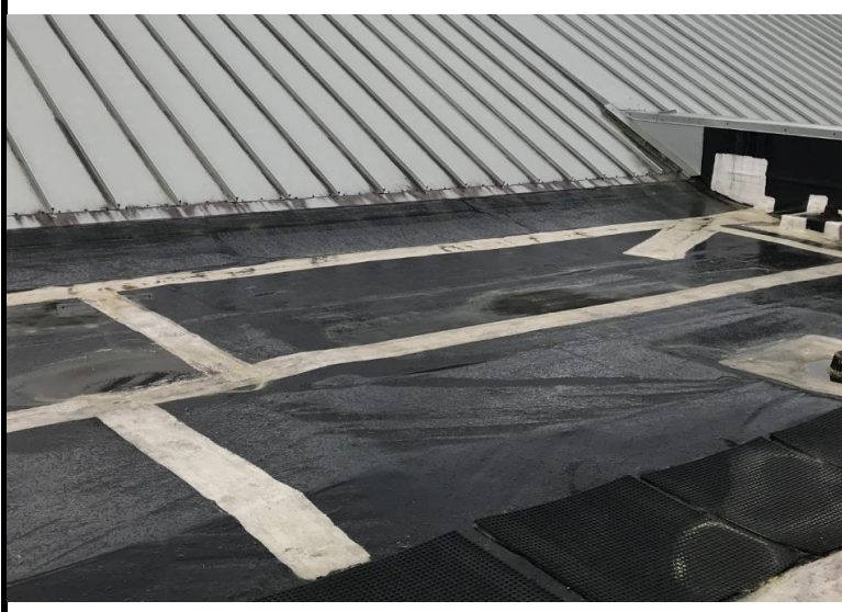
3 Asbestos results were negative for the white roof patch material.
