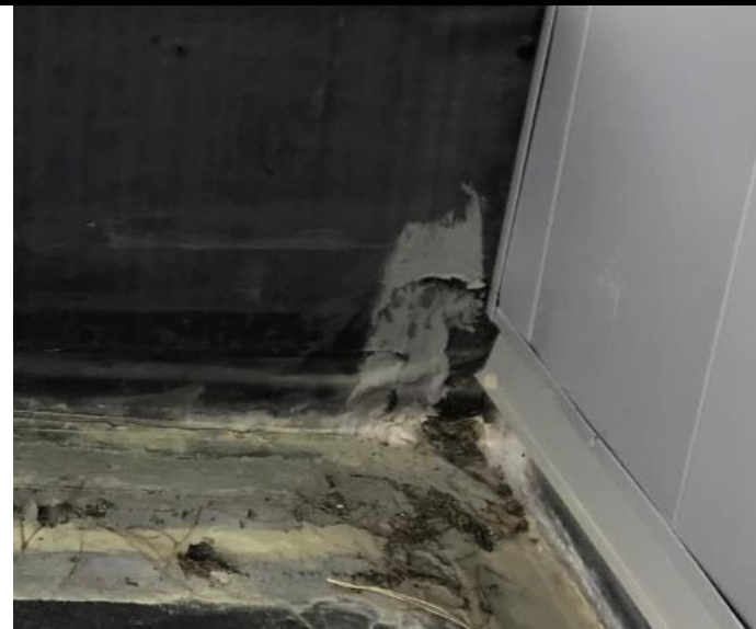
2 Asbestos results were negative for the grey roof patch material.
