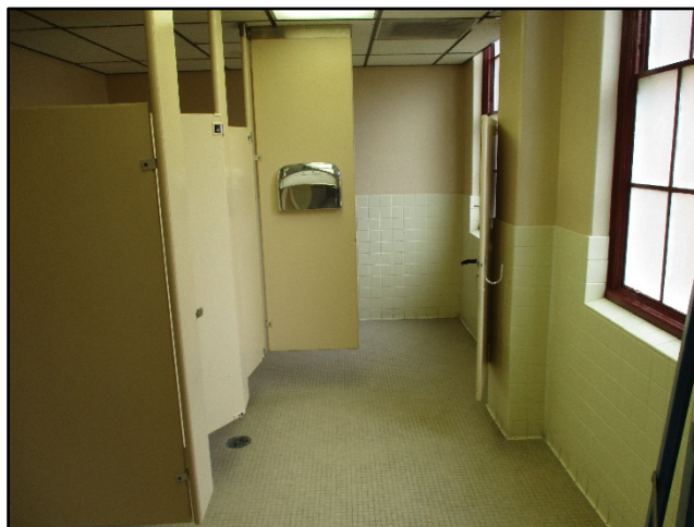
Photo 1. University of South Carolina, School of Medicine Building 1, First Floor Bathroom.
