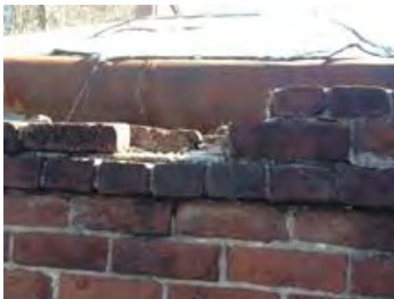
Missing Bricks in Coping on Sumter
