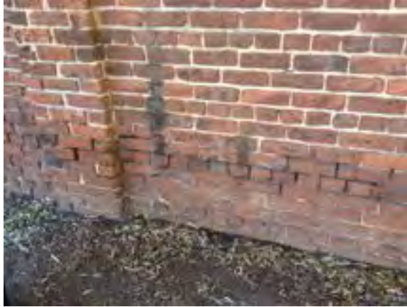
Lower Courses of Wall by Sumter near Pendleton (Note mortar recession in lower wall.)
