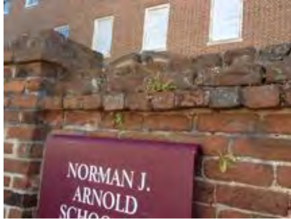
Top Course of Wall by Sumter near Greene (Note mortar recession and vegetation in coping courses.)
