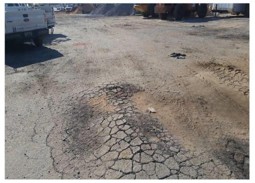
Photo 3: High severity alligator cracks near Boring B-4
