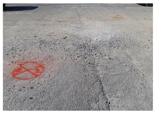
Photo 4: Longitudinal and transverse cracking near Boring B-2
