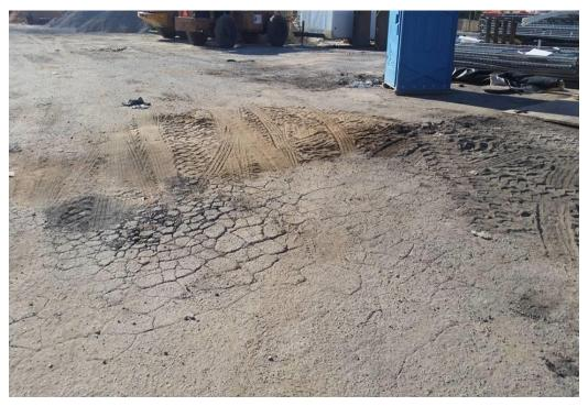
Photo 2: Medium to high severity alligator cracks near Boring B-3
