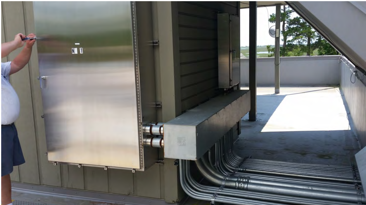
Existing 100 KW electric duct heater and controls to be removed
