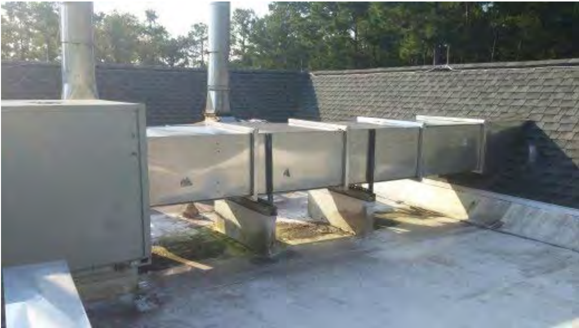
Existing return air and outside air duct to be removed
