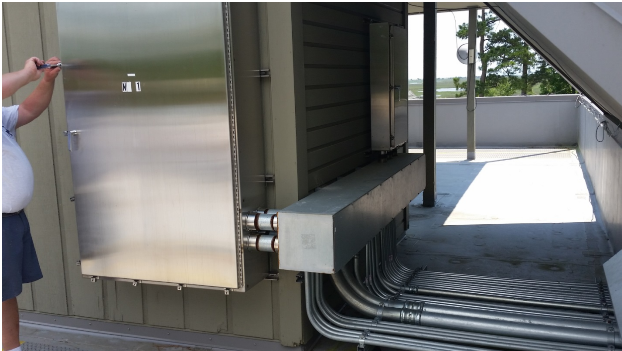
Existing 100 KW electric duct heater and controls to be removed
