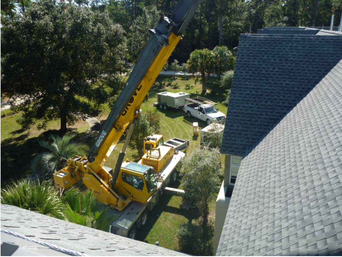
Recent photo showing previous crane removing and replacing HVAC Unit
