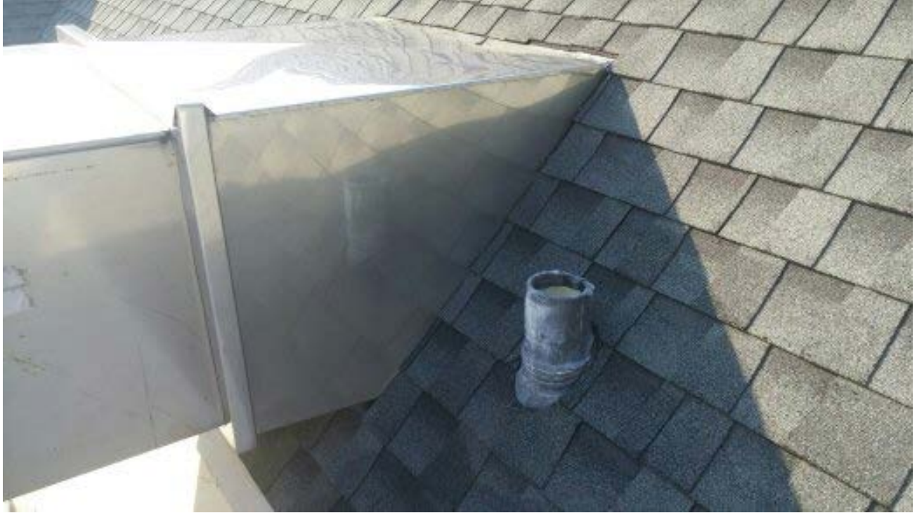
Roof penetration to be closed and roofed over to match existing
