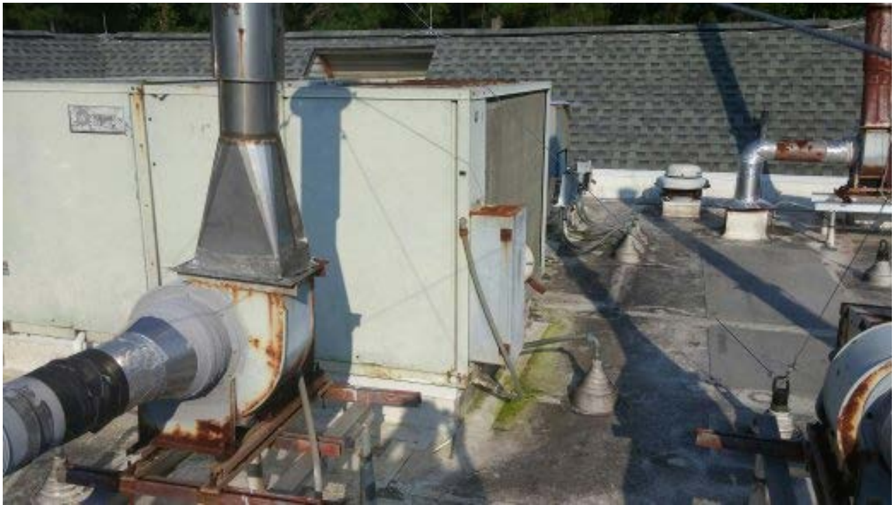
Location of existing electrical power riser thru roof and HVAC unit disconnect switch
