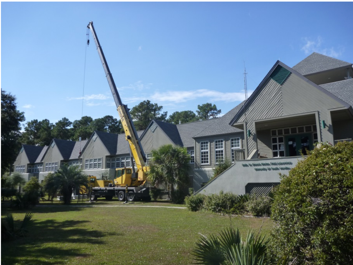
Recent photo showing previous crane removing and replacing adjacent HVAC Unit
