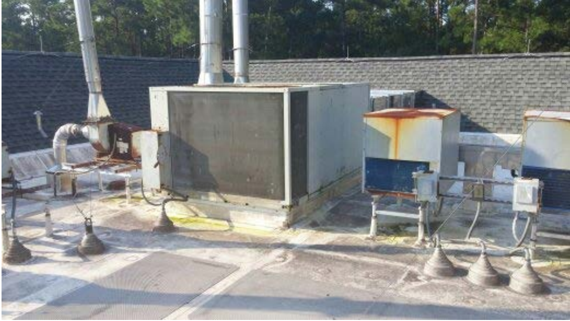
Existing 15 ton to be removed and replaced with new 12 ton HVAC unit
