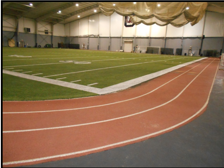
1 General view of the subject athletic track and practice field area to be demolished.
