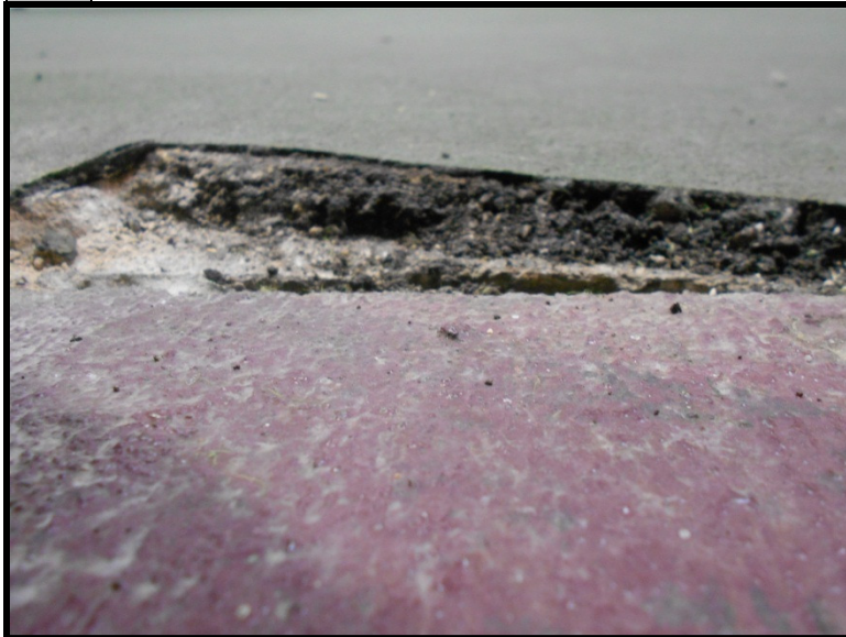
7 Black and green tennis court surface material. Both black and green layers are to be removed.
