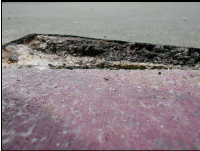
7 Black and green tennis court surface material. Both black and green layers are to be removed.
