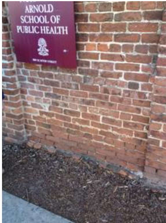
Lower Courses of Wall by Sumter near Greene (Note mortar recession in lower wall.)
