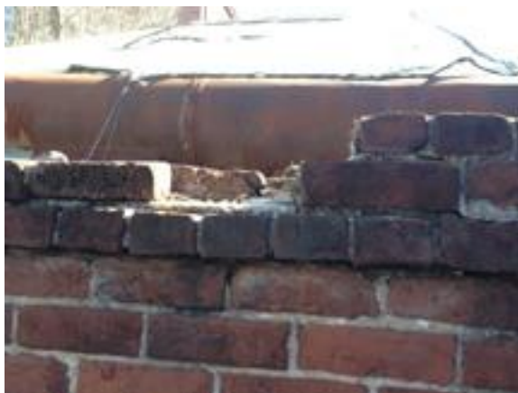
Missing Bricks in Coping on Sumter
