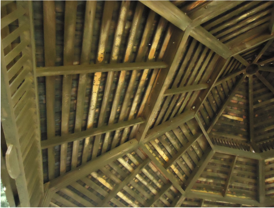
IMAGE 2-A : An area in need of repair on hand rails
