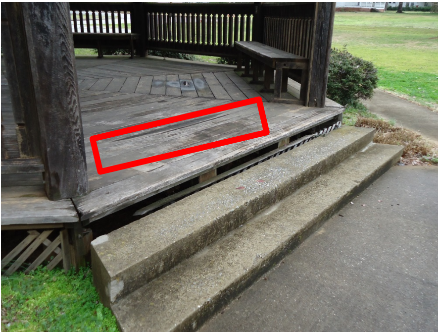
IMAGE 2-E : Area of floor in which sponginess was observed (outlined in red)
