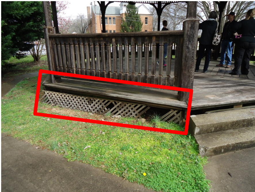
IMAGE 2-I : Example of foundation skirting lattice in need of replacement
