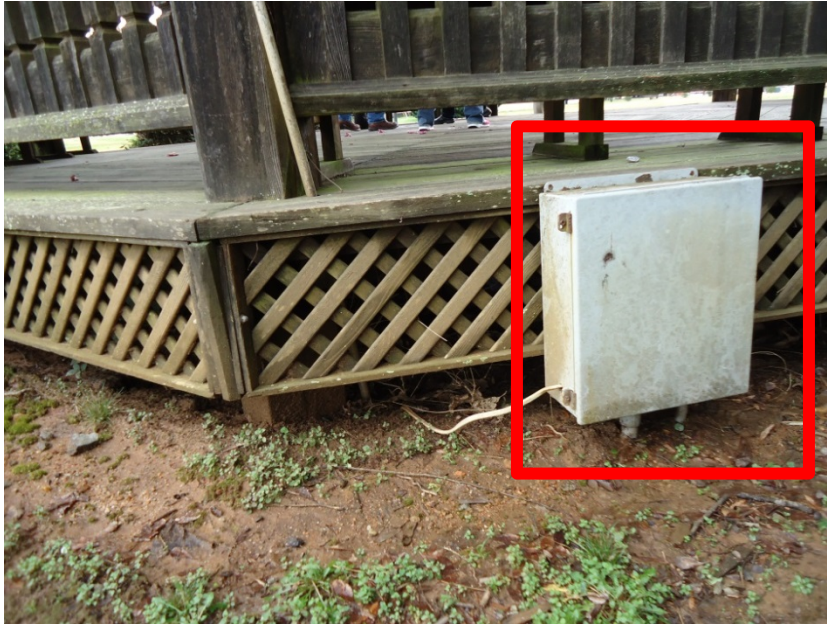
IMAGE 3-B : Area of exposed Romex wire and damaged conduit
