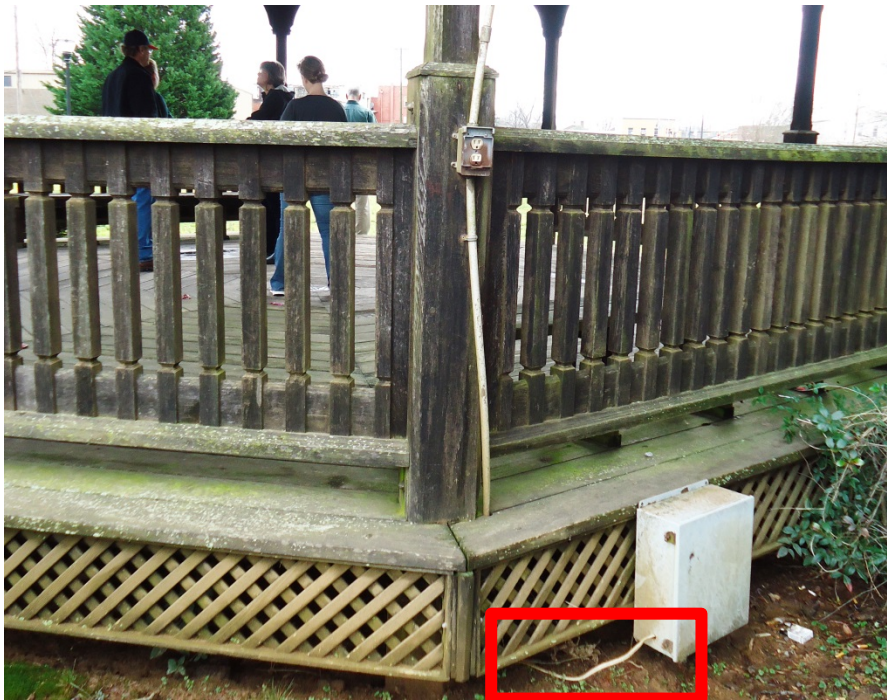
IMAGE 3-B : Area of exposed Romex wire and damaged conduit
