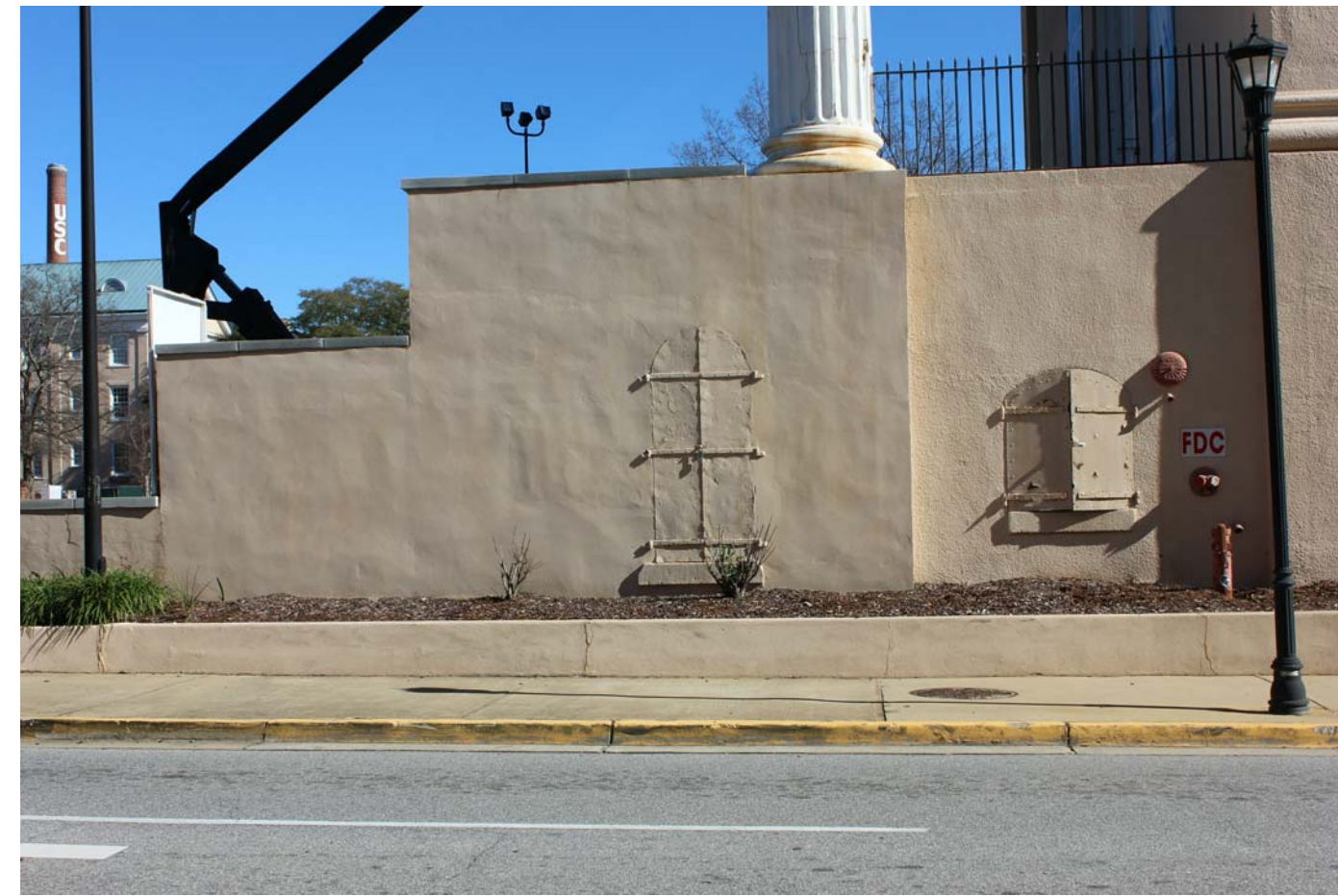
WEST ELEVATION PHOTO 2- EXISTING PLANTER WALL
