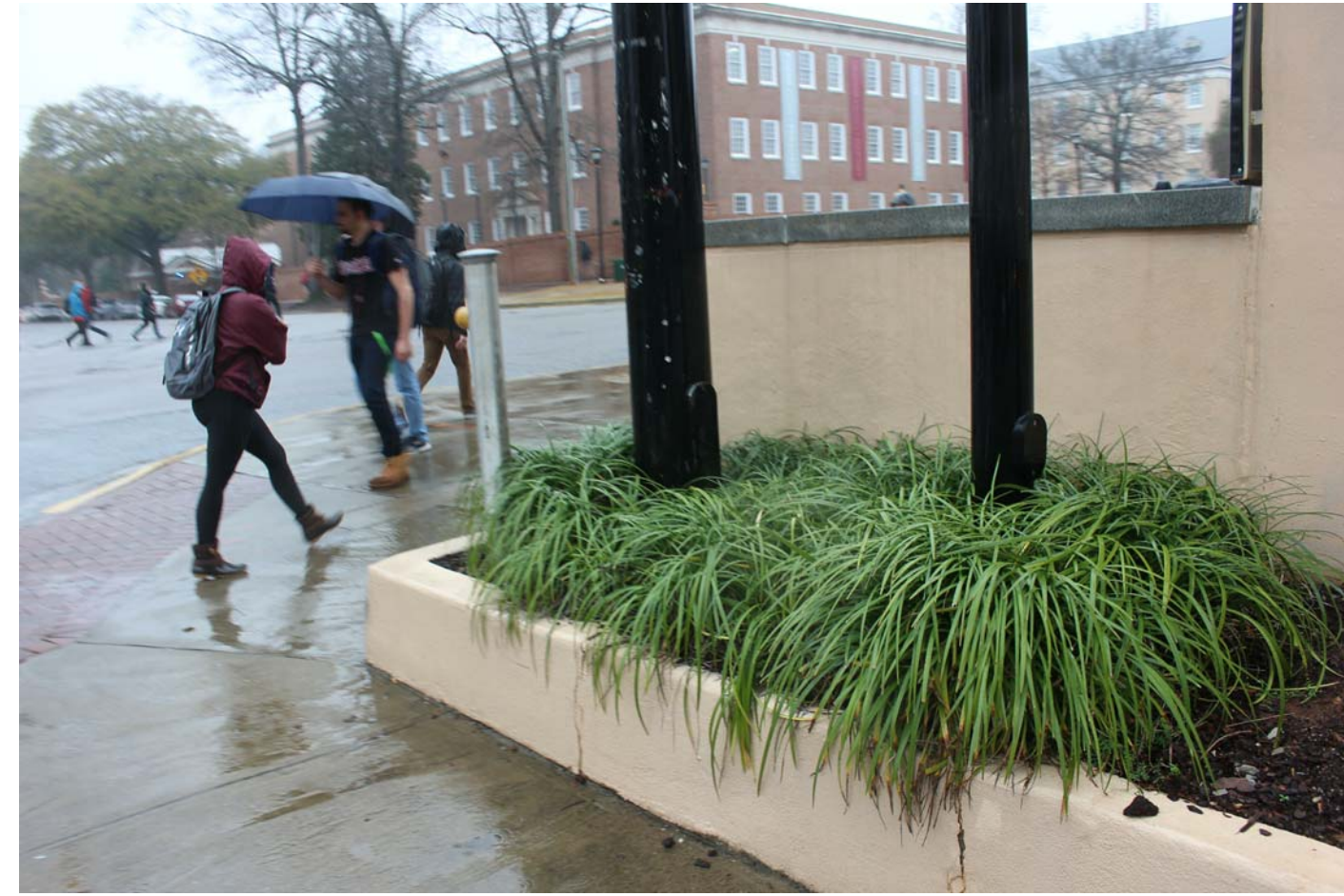
WEST ELEVATION PHOTO 1- EXISTING PLANTER WALL
