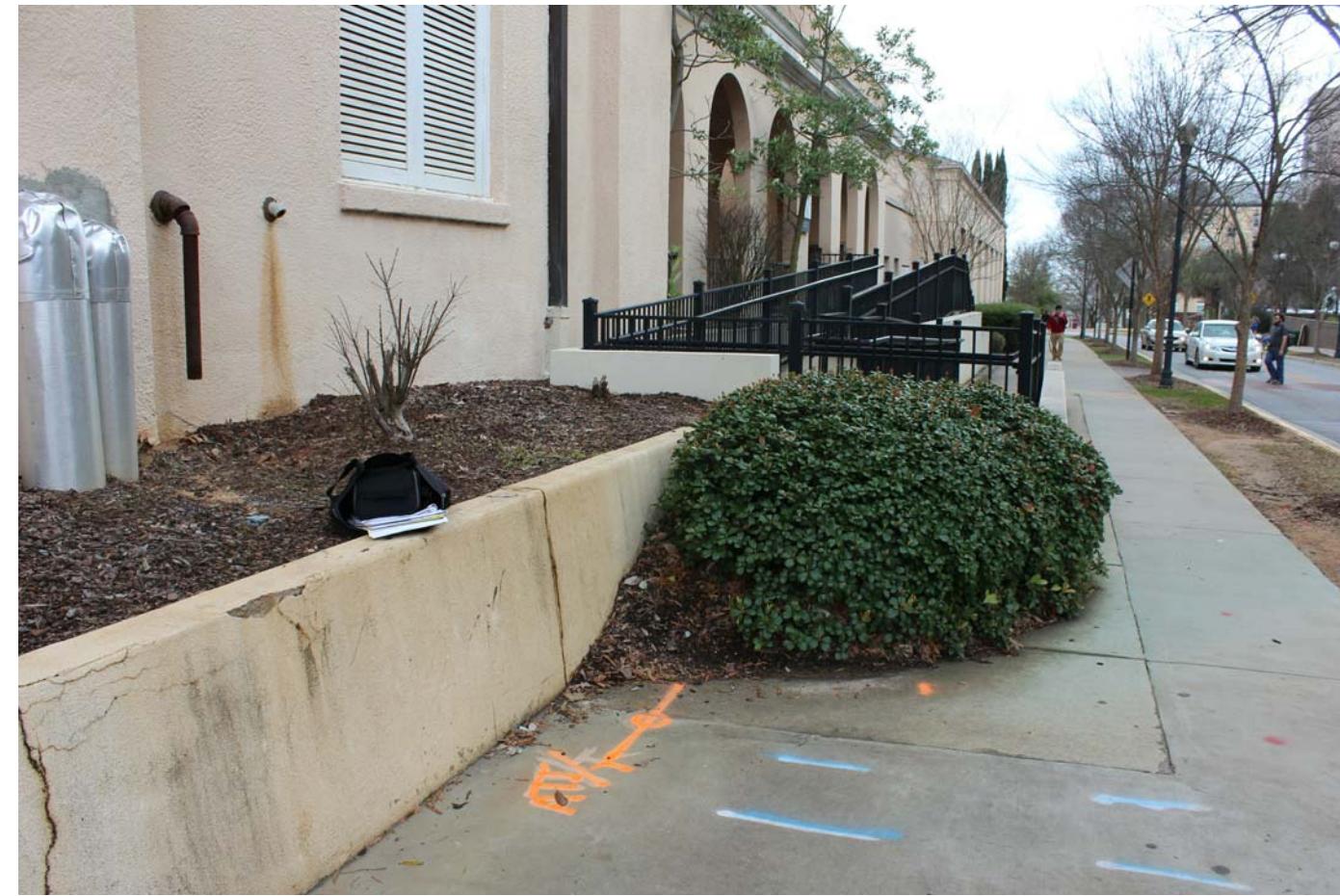
WEST ELEVATION PHOTO 4- EXISTING PLANTER WALL
