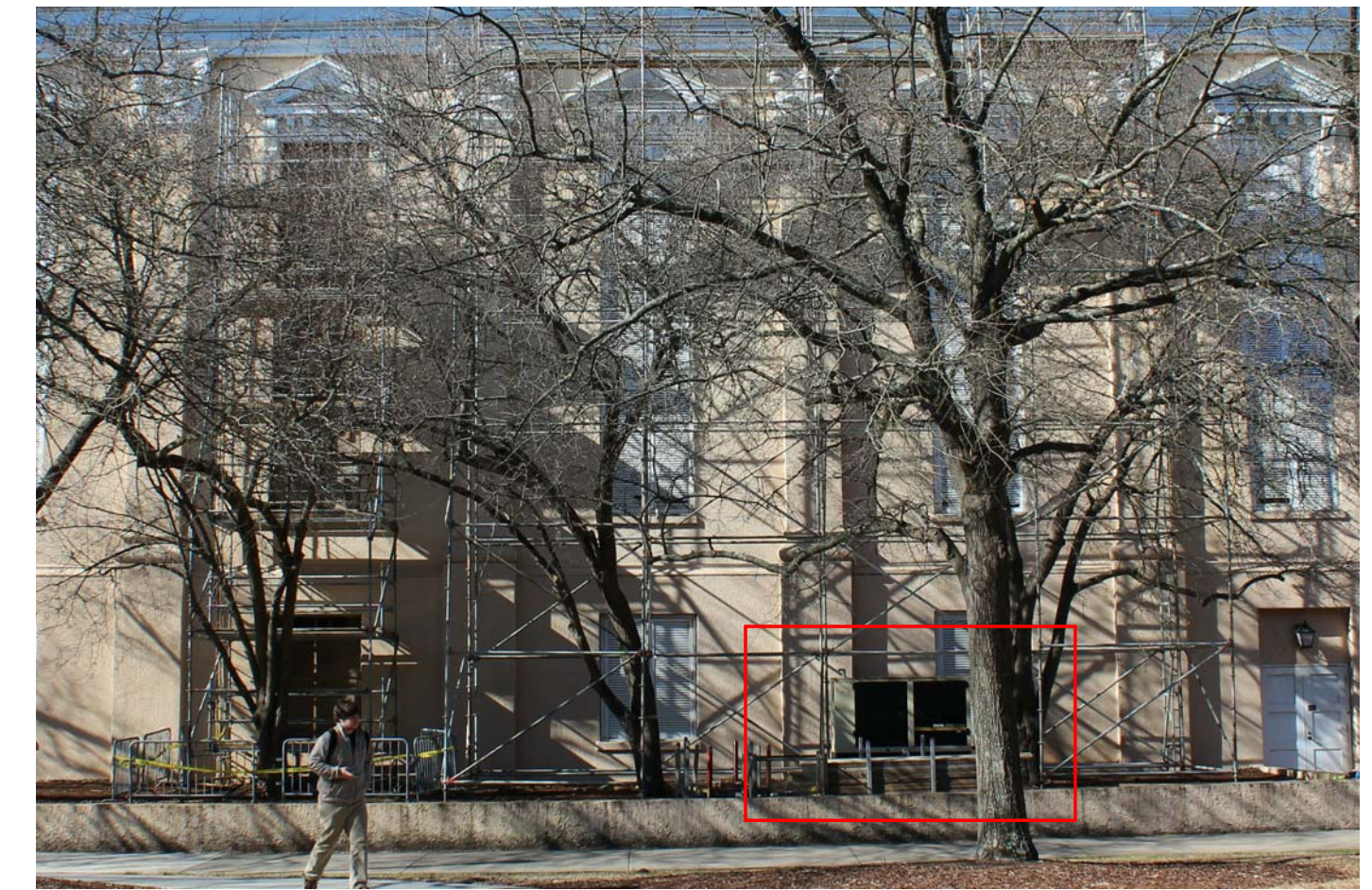
EAST ELEVATION PHOTO- EXISTING PLANTER WALL AND GENERATOR
