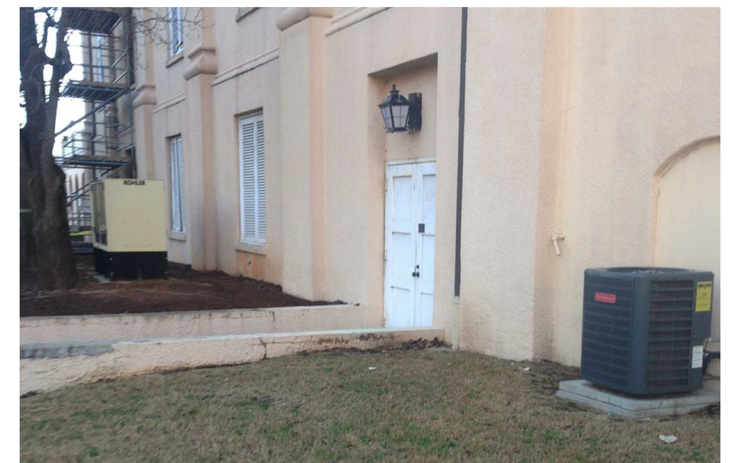
EAST ELEVATION PHOTO- EXISTING GENERATOR AND CONCRETE PAD
