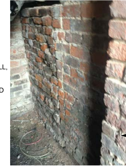
MASONRY WALLS UNDER STAIRS
