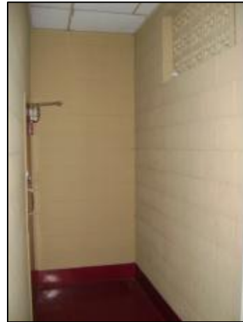
View into Men's Restroom Entrance
