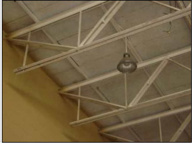
View of roof joists
