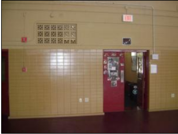
View of glazed brick and honeycomb vent
