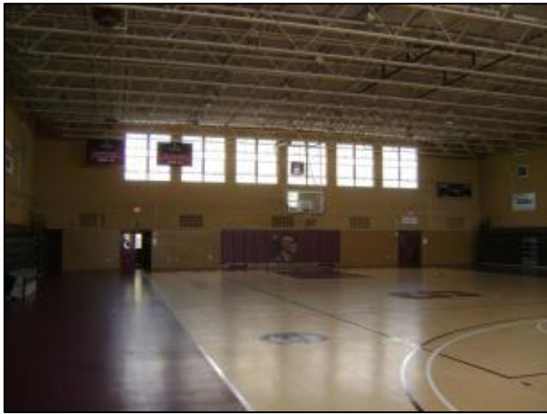
South Wall of Gym
