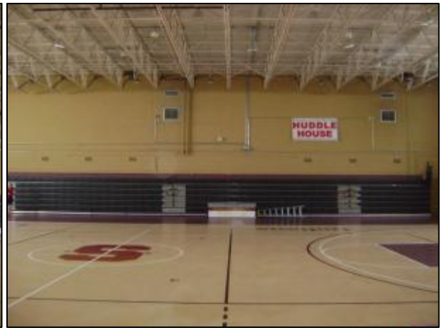
East Wall of Gym
