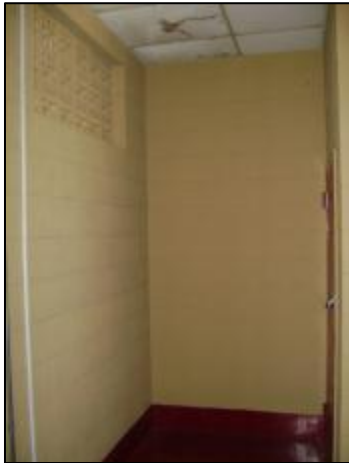
Interior View into Women's Restroom Entrance
