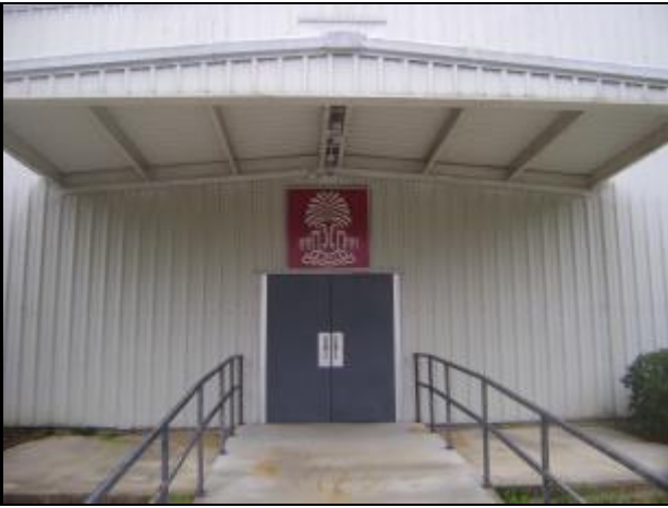
Left Covered Entrance
