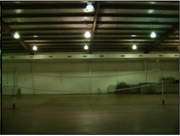
Assembly Area looking Northwest
