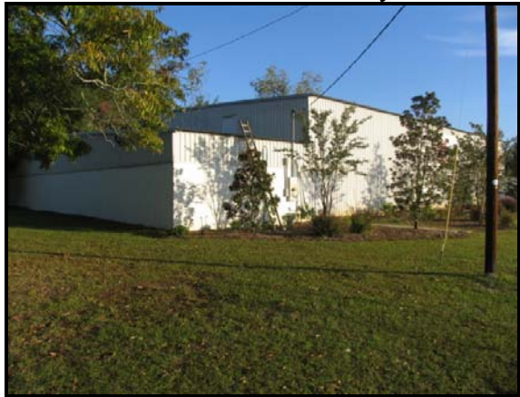
Southwest Side of Facility
