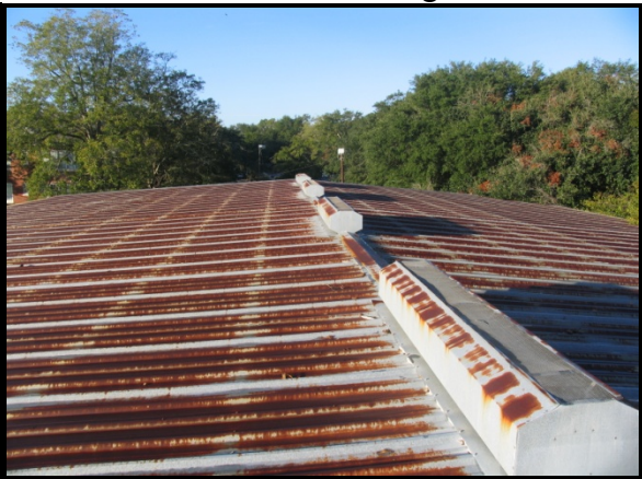
Main Roof View Looking West
