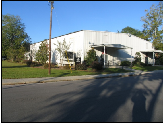
Southeast Side of Facility
