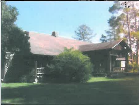
Hut Front View
