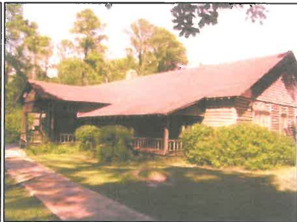
Hut Front-Side View
