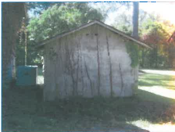
Storage Building Rear Elevation
