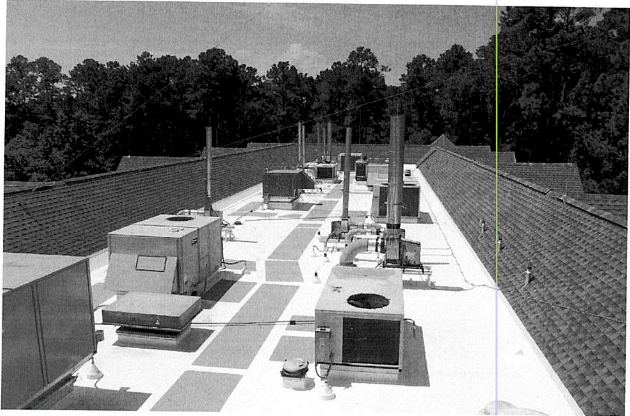
Aerial view of existing units within mechanical well of marine lab. Notice new membrane roof system.
