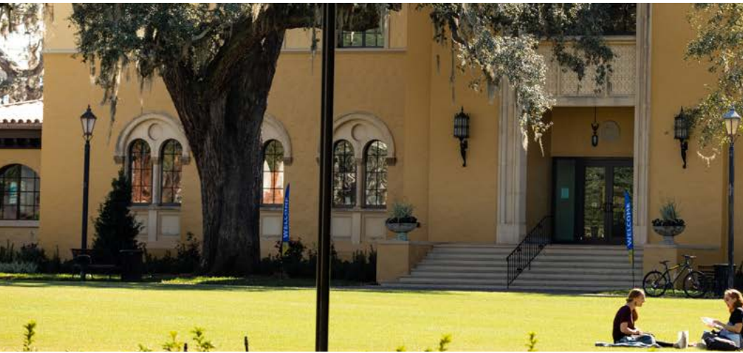
Located at the center of Rollins College's campus in Orlando, the Kathleen W. Rollins Hall is being renovated to house academic and student affairs programs, including the career center. (Photo by Scott Cook)
