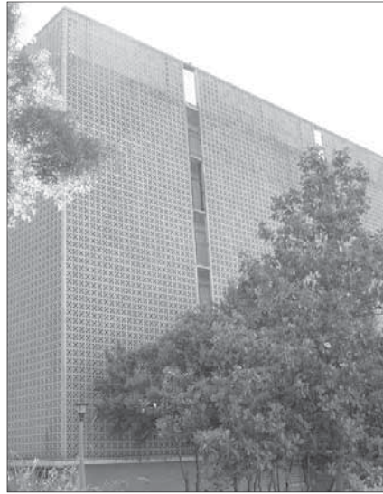
The towers will be demolished this summer.
