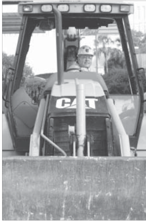
New Horizon As part of the Sept. 15 rollout of the research campus' new name, President Sorensen dons a hardhat and drives a front-end loader on the site of what will become the Horizon Center on Blossom and Assembly streets.
