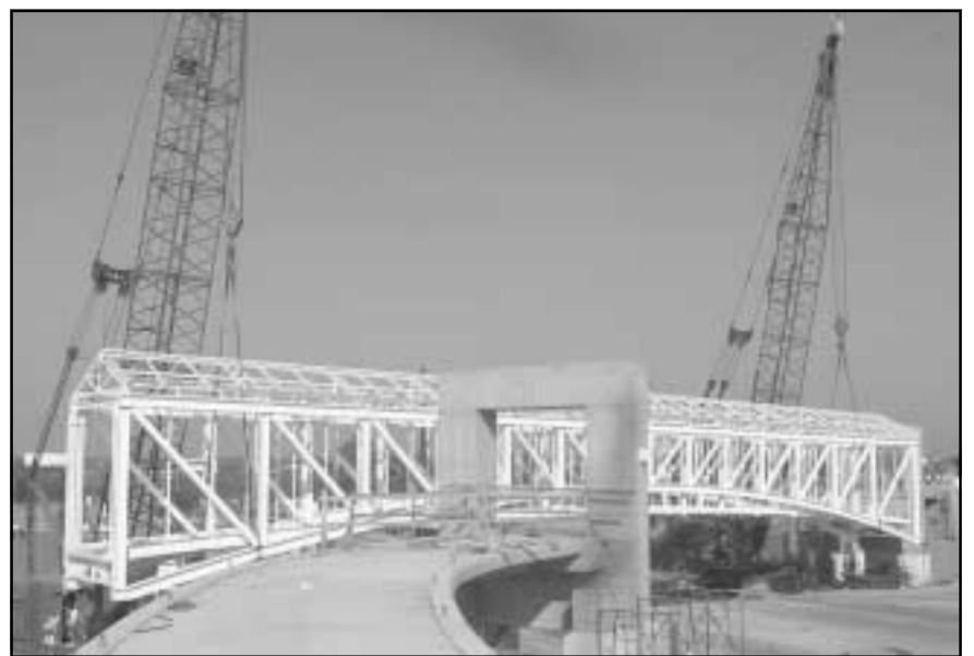
Cranes lift the new pedestrian bridge over Blossom Street.
